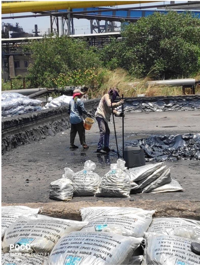
Figure 1 Pitch Cutting in Progress
