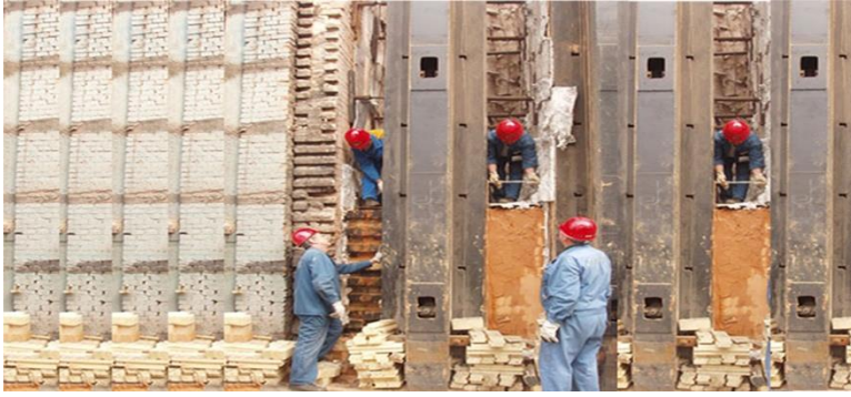
Work under progress
