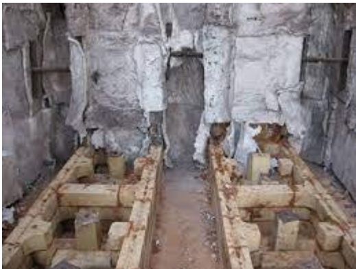
Refractory fitting under progress: ambient temp 50 to 60 deg C. (Fig-5)
