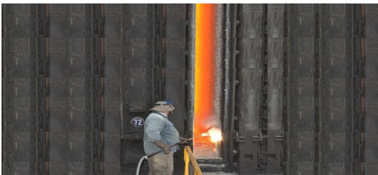
Battery from coke end after removing door Temp: 1050 degree centigrade (Fig-2)
